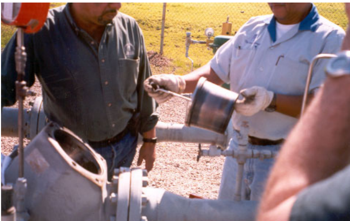
Figure 6.0 - Top Entry Design of Model 900TE Flexflo® Regulator Allows Easy In-Line Maintenance
