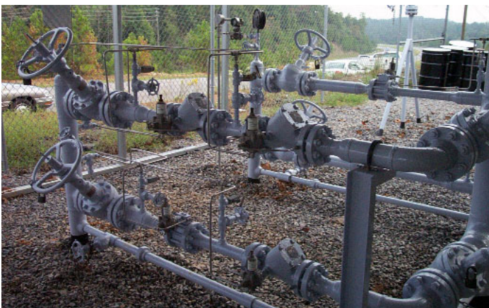
Figure 8.0 - Model 900TE Flexflo® Power Plant "Startup" Regulator with Flow Control Override
