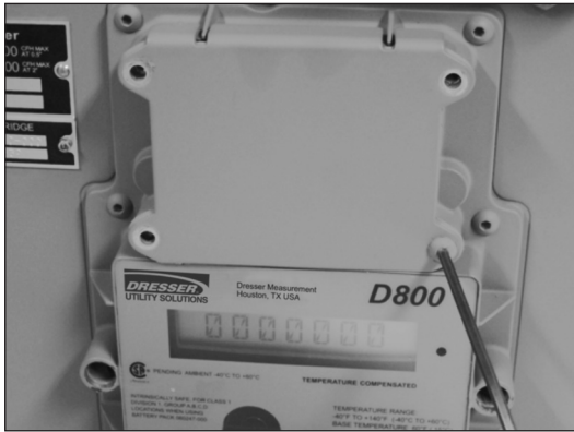
Figure 9.7 - Remove 4 screws on battery compartment
