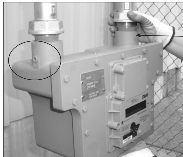
Figure 11.1 - Differential pressure taps are located on the inlet and outlet connectors
