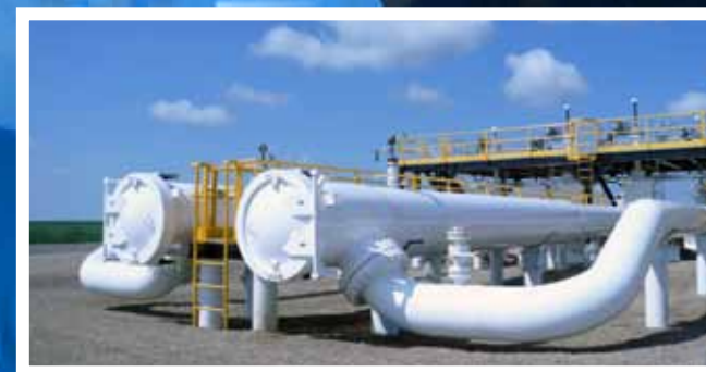
YOKE STYLE QUICK OPENING CLOSURES (QOC)
